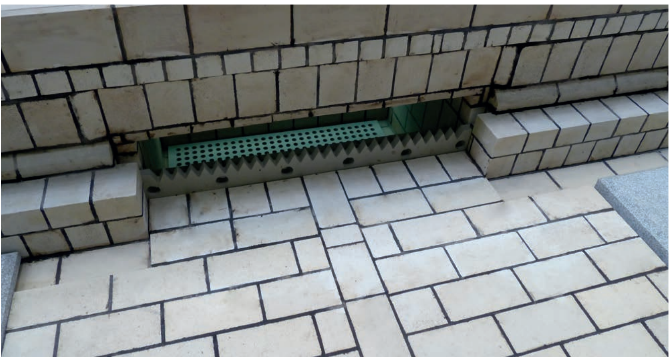
Brick lining with CHEMOKITT FU 1310
