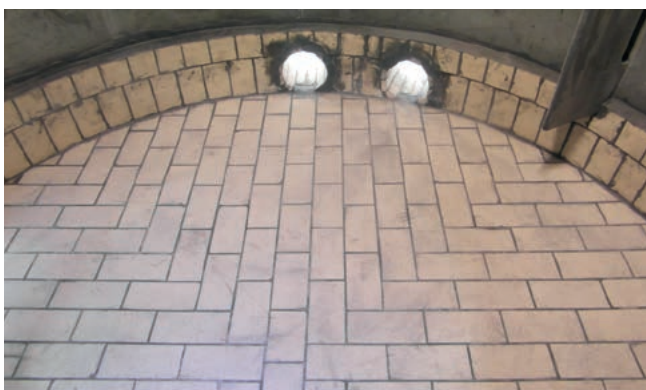
Brick lining a tank floor with Asplit CN
